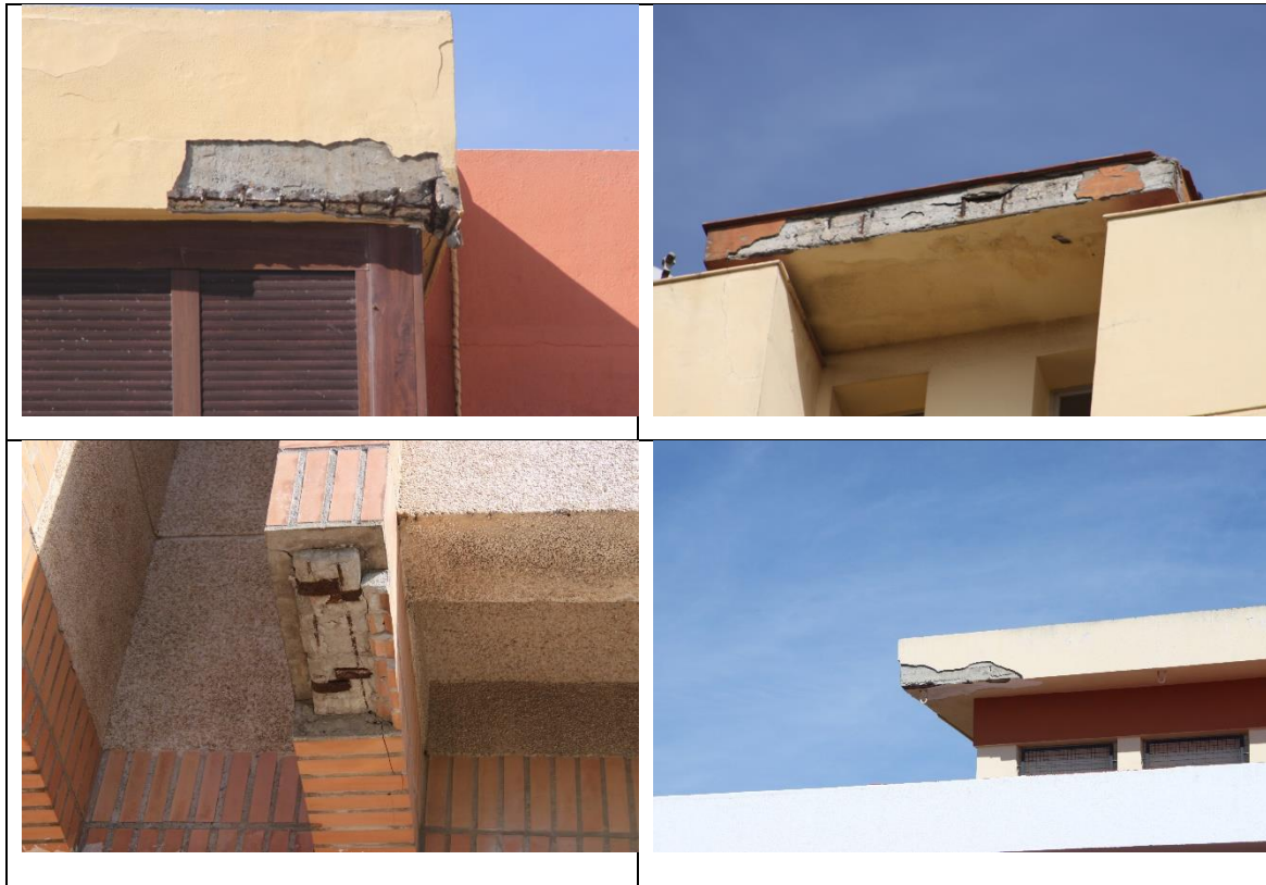
Figure 2. Pathologies observed in buildings located in the Mediterranean coast: Inadequate cement type and low concrete cover
